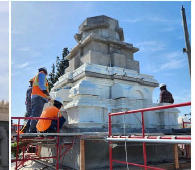
GFRC Work, Concord, California
